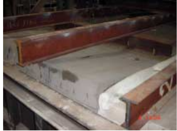
Solid slab Phase 2 at 80 min. Deflection and support.
