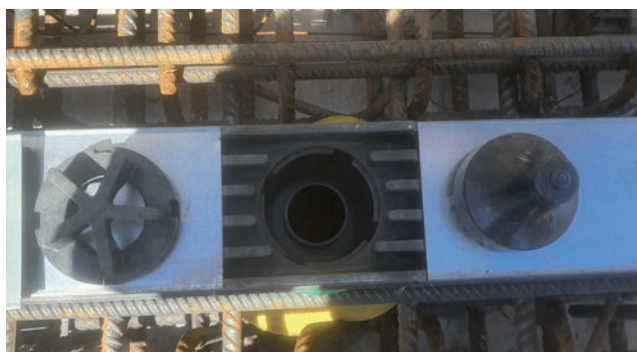
Straight intake filter with detachable inspection flap and drain connection NW 125 or NW 100.
