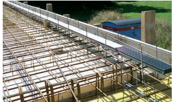
Installation with gutter elevation
